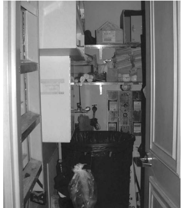
FIGURE 11.11 A typical public area utility closet at the Bellagio. Note the chemical mixing station at the rear of the closet. (Photo courtesy of Bellagio, MGM Mirage™, Las Vegas, Nevada.)
