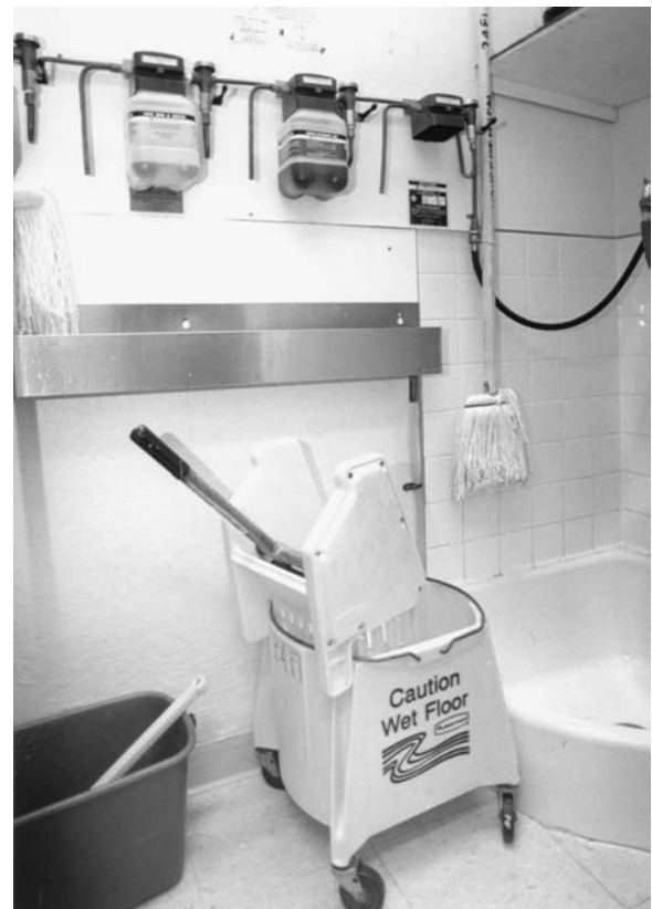
FIGURE 10.45 Another chemical mixing station located near a mop sink in a satellite storeroom, allowing users easy access. Note the labeling of containers, required by Hazardous Communications Laws (HazComm). Information regarding hazards connected with a product must be clearly specified on the container. Products in smaller containers must carry the same precautions as the container from which the product was drawn. (Photo courtesy of MGM Mirage.)
