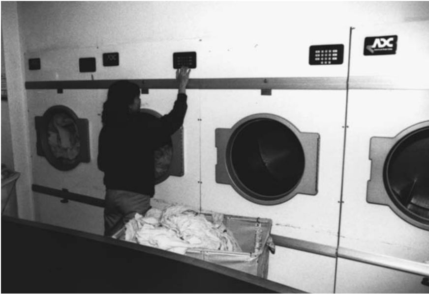
FIGURE 15.25 Four 100-pound dryers make a compatible arrangement with four 50-pound washers. (Photo taken with permission.)
