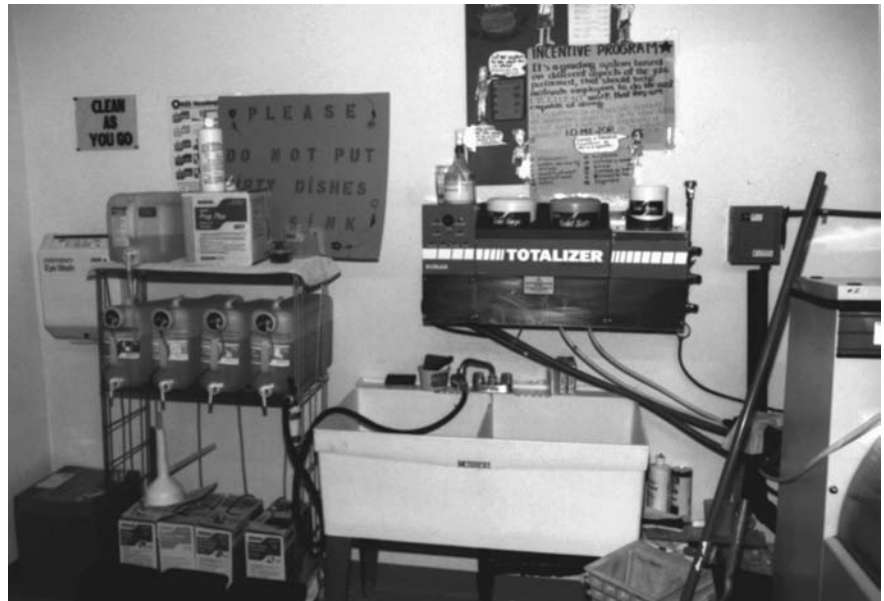
FIGURE 15.27 Soak sink and chemical mixing center. Note detergent lines leading to washing machines. Other chemicals are arranged for proper dispensing. (Photo taken with permission.)
