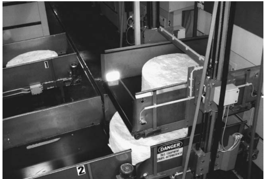
FIGURE 15.6 The cake is transported automatically via a conveyor to a lift that picks up two cakes at a time and moves them to a dryer. (Photograph courtesy of Mission Industries, Las Vegas.)
