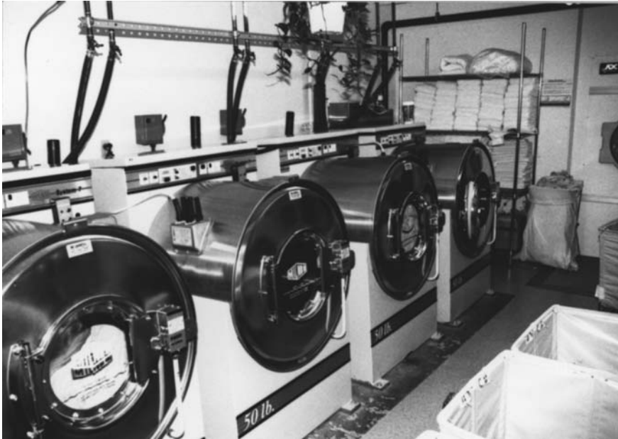
FIGURE 15.24 A bank of four 50-pound washers plumbed for automatic chemical and water intake. (Photo taken with permission.)
